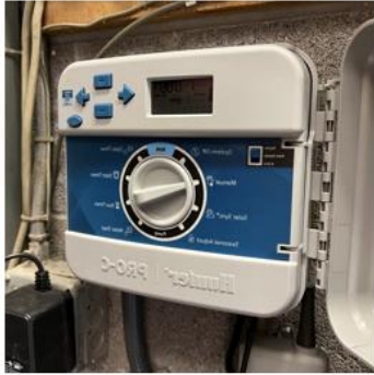
Installed new irrigation system
