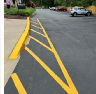
Resurfaced & restriped the parking lot
