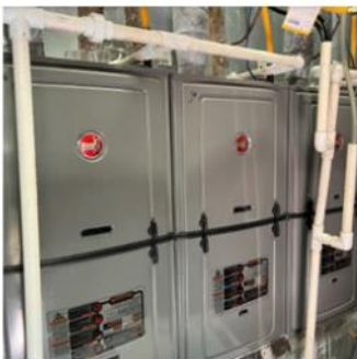
Replaced 4 furnaces serving the Sanctuary
